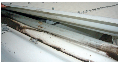
Photo : © SARETEC - Pierre LAMORIL
