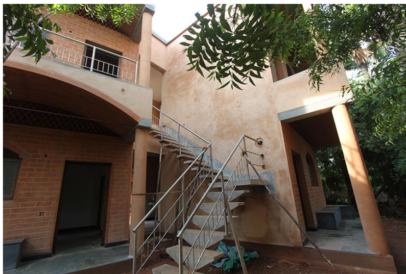
Figure 5: Sharanam Center for Rural Development - Phase II, Auroville Earth Institute, Inde
