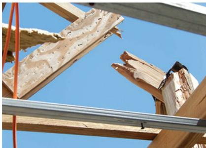
Figure 2 : Section insuffisante
