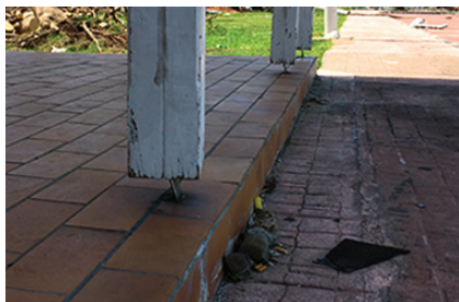
Figure 5: Post base bending
