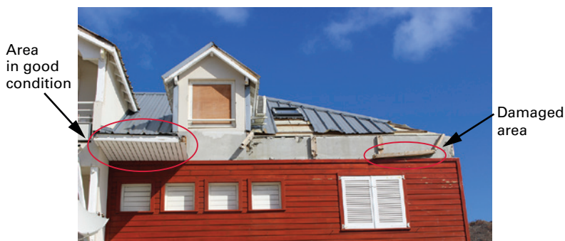
Figure 4: Undersized eave
