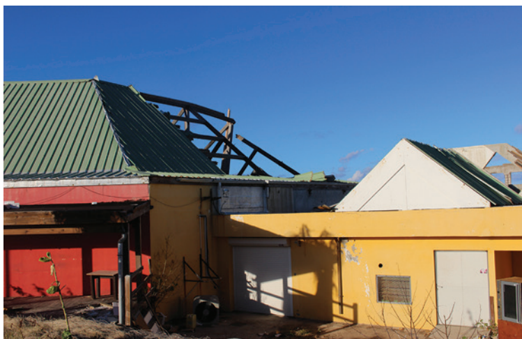
Figure 5: Incorrectly braced frame
