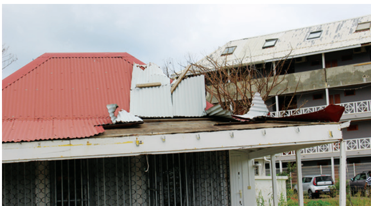
Figure 6: Uplift of the roof edge – sheet too thin and insufficiently steep, insufficient fastening causing perforation
