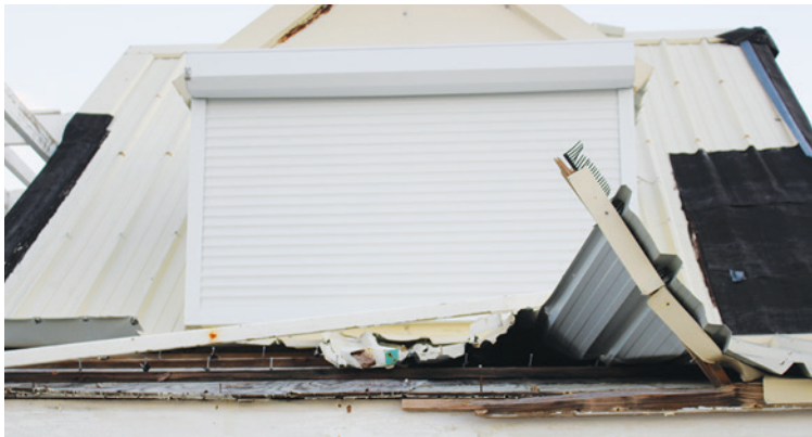
Figure 3: Batten with cross section that is too small and/or is fastened insufficiently
