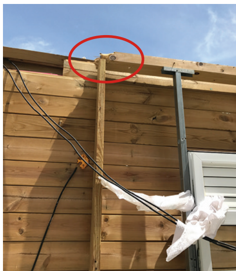
Figure 1: Cross-section probably not substantial enough (CAUE)
