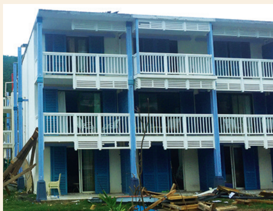
Figure 2: Louvred shutters that provided good protection
