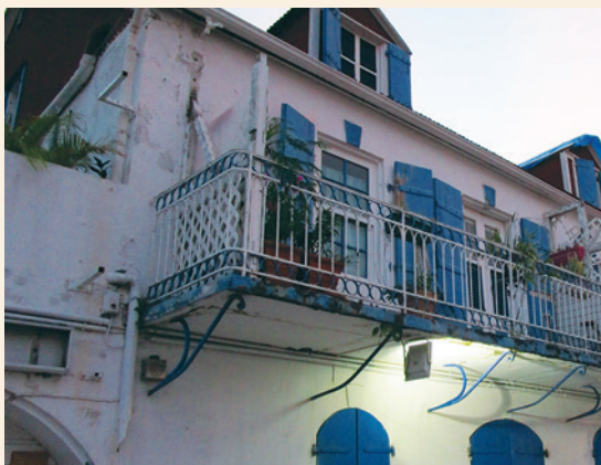
Figure 1: Opaque shutters that provided good protection
