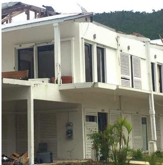
Figure 3: Insufficiently-attached shutters
